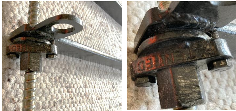
Figure 4. Anchor nut and steel strip with a hole for strap attachment
